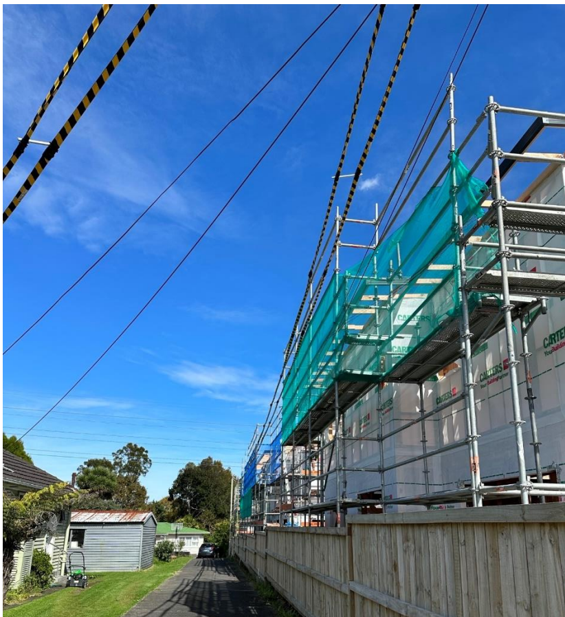
Figure 3: Non-compliant building and scaffold near 400V lines. Unauthorised third-party insulation was applied by an unknown person. Source: Vector.
