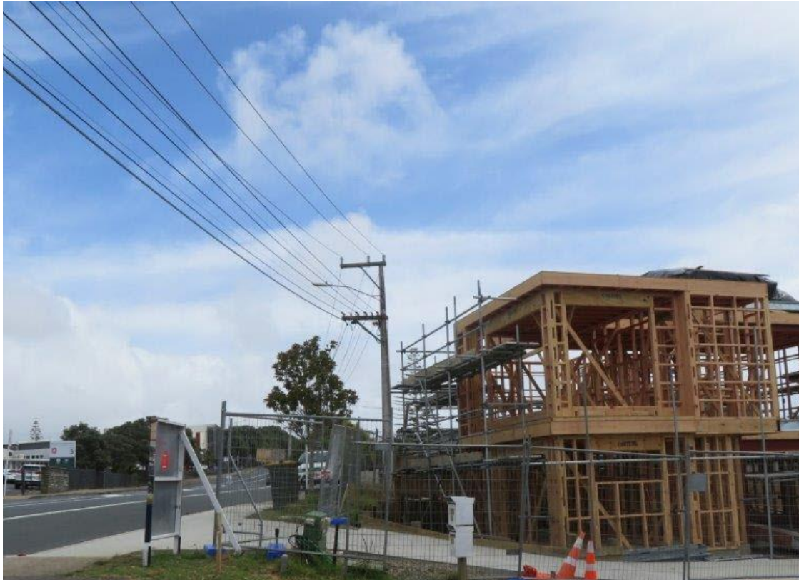
Figure 1: Non-compliant building and scaffold near 400V and 11kV lines – the building had to be partially demolished and re-consented to compliance. Source: Vector.
