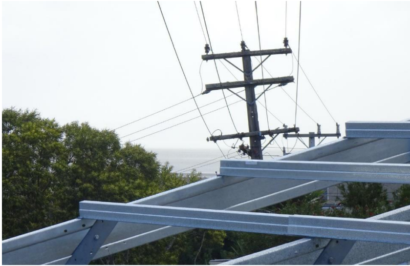
Figure 2: Non-compliant rural building below 400v and 11 kV lines. Source: Vector.
